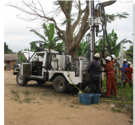
Drill Rig, Angola
