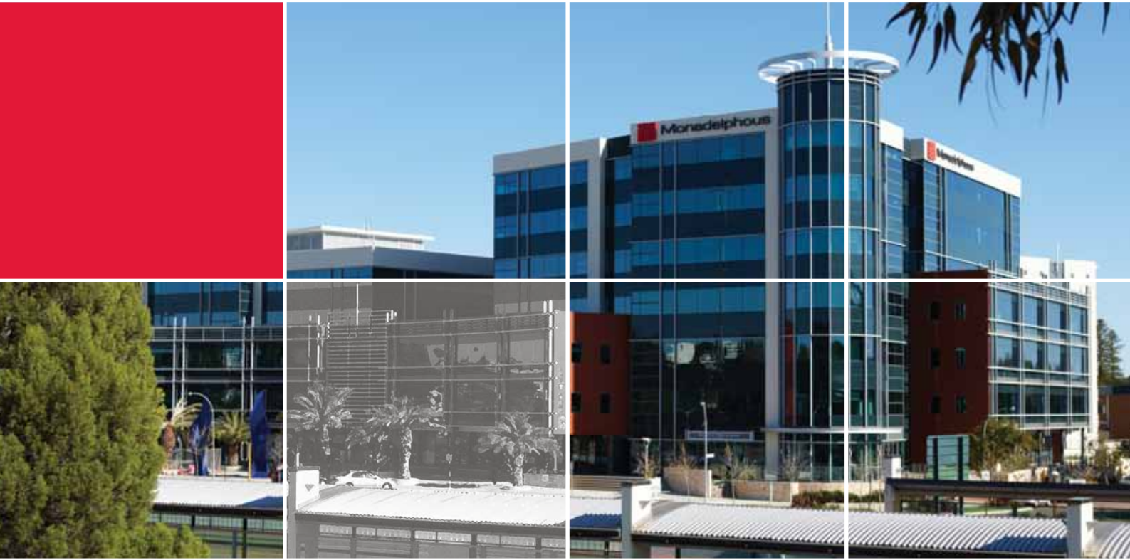
Monadelphous head office at 59 Albany Highway, Victoria Park, Perth (WA)
