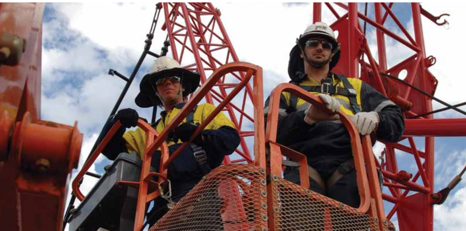
Monadelphous at Woodside's Pluto LNG Project, Karratha (WA)
