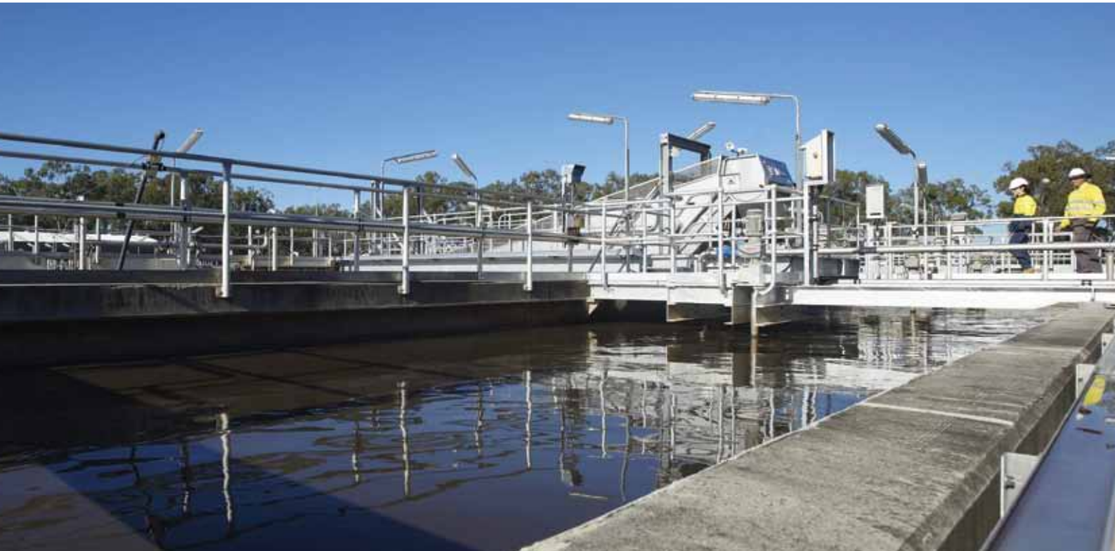
Monadelphous at Unitywater's Burpengary East Sewage Treatment Plant Upgrade (Qld)
