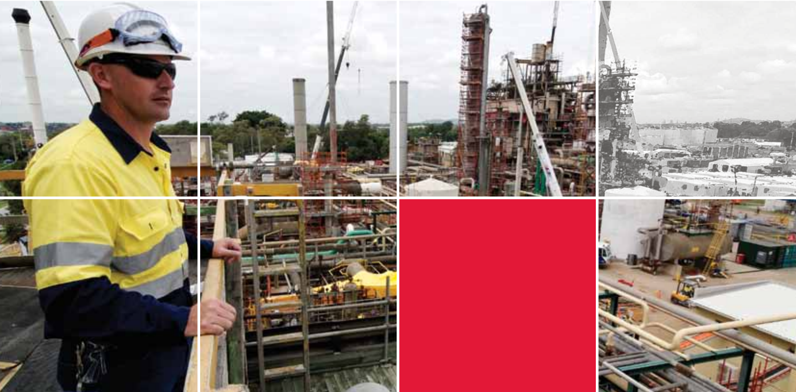
Monadelphous at Incitec Pivot Limited, Gibson Island (Qld)
