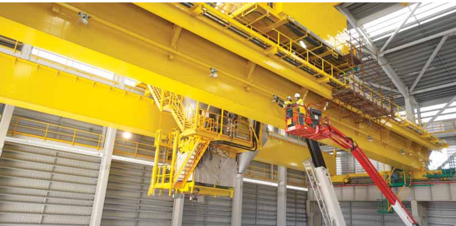
Monadelphous at Boyne Smelter's Carbon Bake Furnace 4 Project, Boyne Island (Qld)
