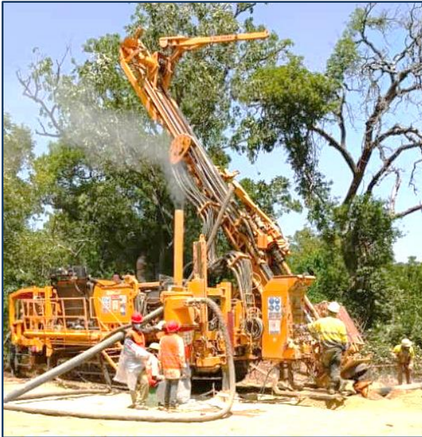
Figure 4 | RC drilling in September quarter at Ferke
