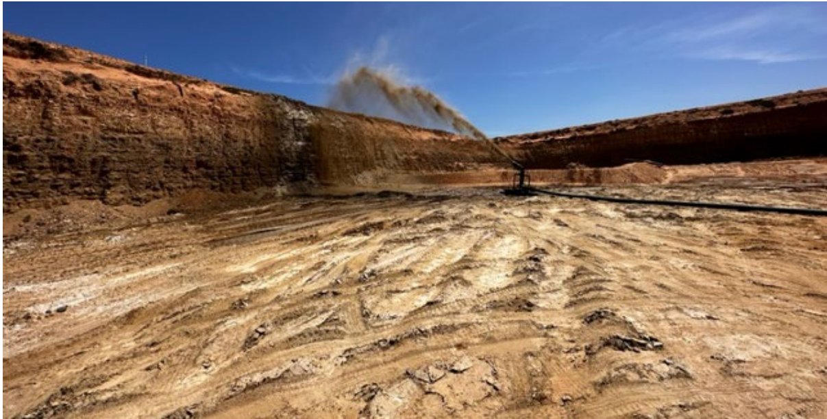
Figure 2 Initial tests with slimes spray gun - being used to seal the floor and walls of the mining pit with low permeability thickened slimes
