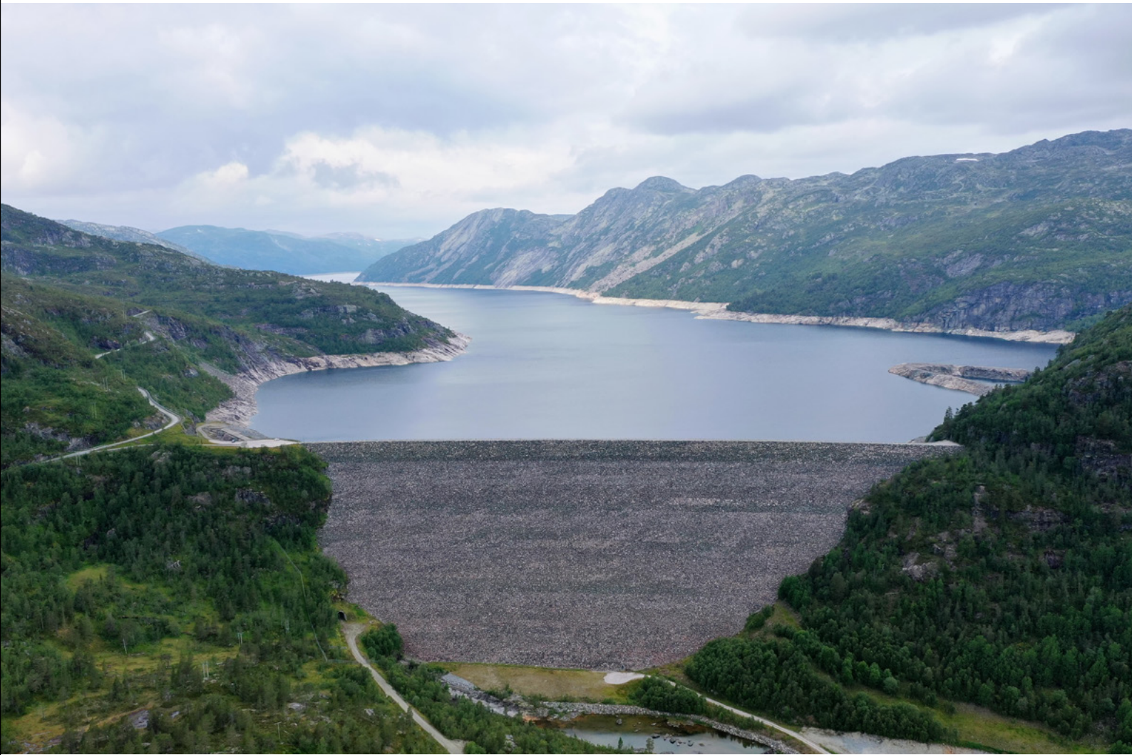
Holen pumped storage power plant, Norway (Otra Kraft).
