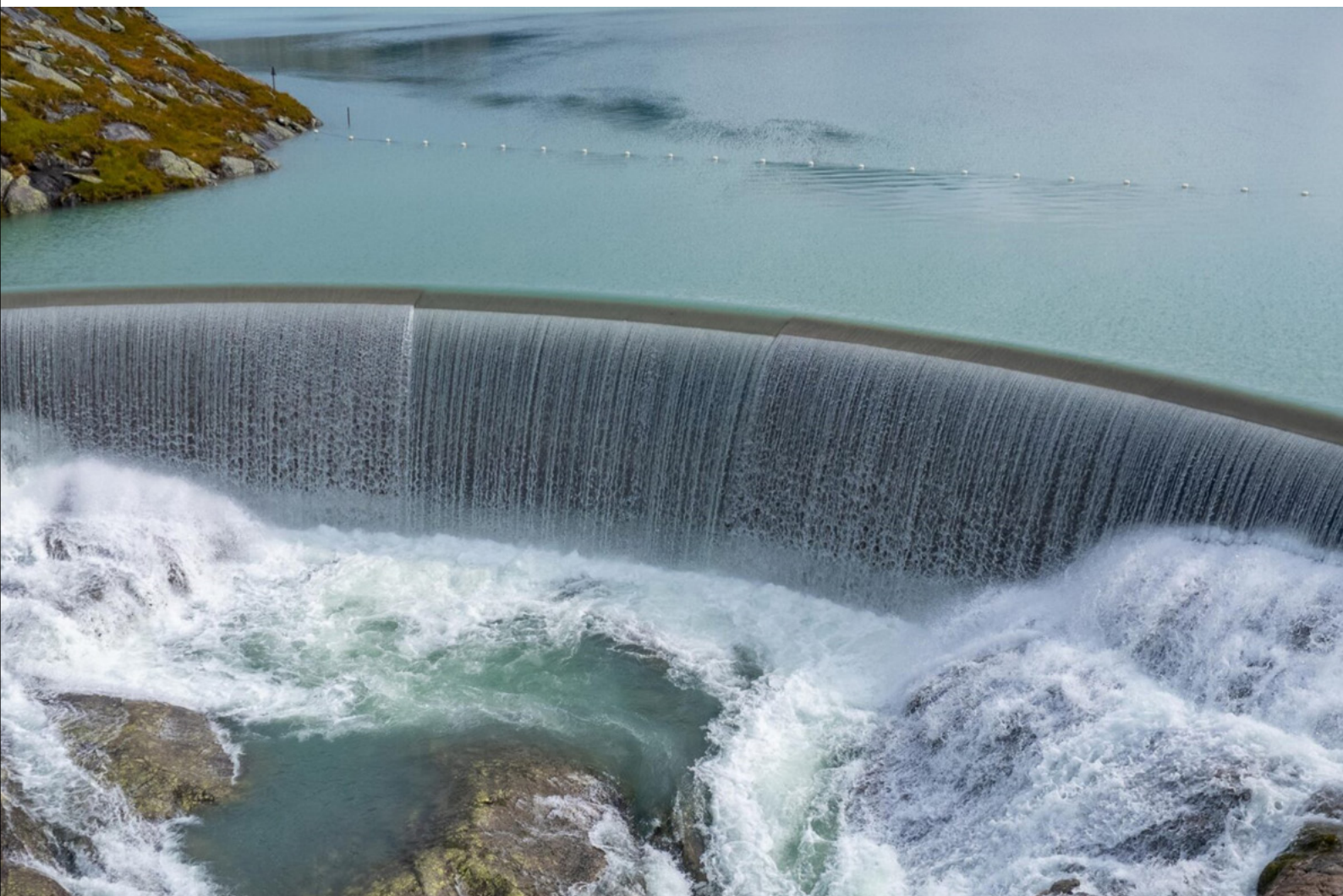
Bláfalli Fjellhaugen power plant | Photo: Magne Langaker
