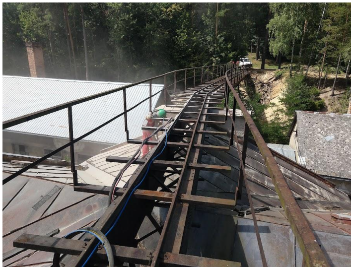
Image 3 (left): cleaning and painting the rail link bridge over the engine room; Image 4 (right): near complete roof repairs and installation on the engine room at the Sturec project;
