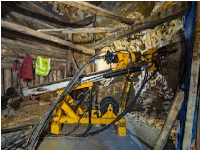
Fig 1: Drilling first 5 holes from Chamber One
