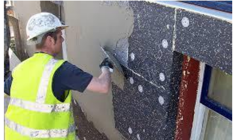
Installing flame retardant insulation foam
