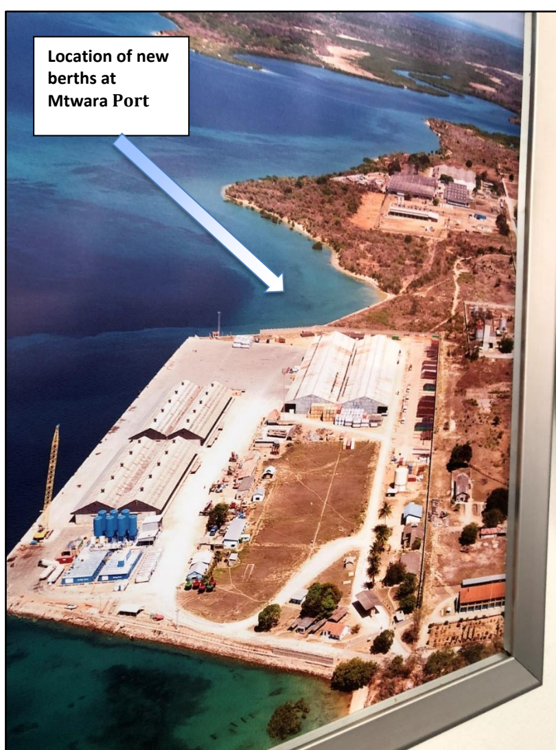
Figure 2: Aerial view of Mtwara Port
