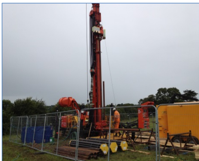
Figure 3: Priority Drilling - Hanjin D&B35 Drilling Rig
