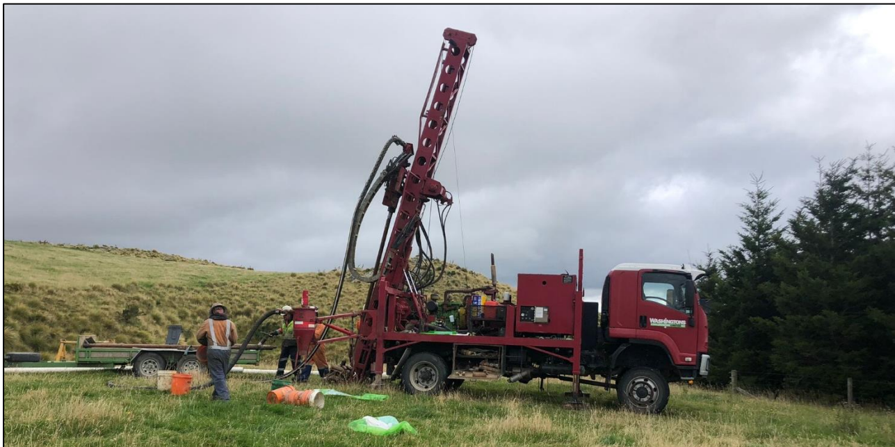
Figure 1 Drilling rig on site at Lammerlaw
