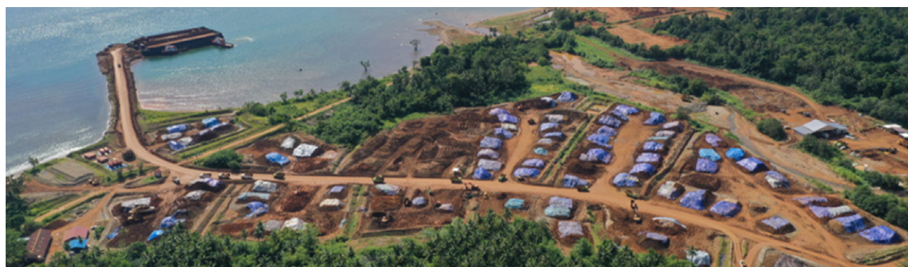
Stockpiles and jetty operating at 2.5m tpa
