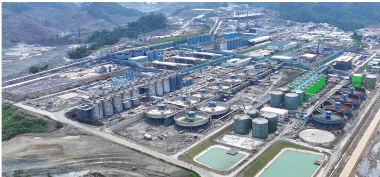
ENC HPAL Smelter construction progress
