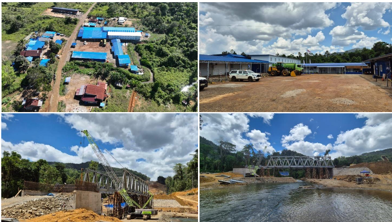
Sampala Mine camp and bridge construction
