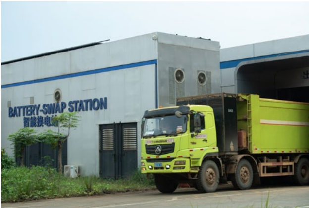
EV battery swap station and electric loader
