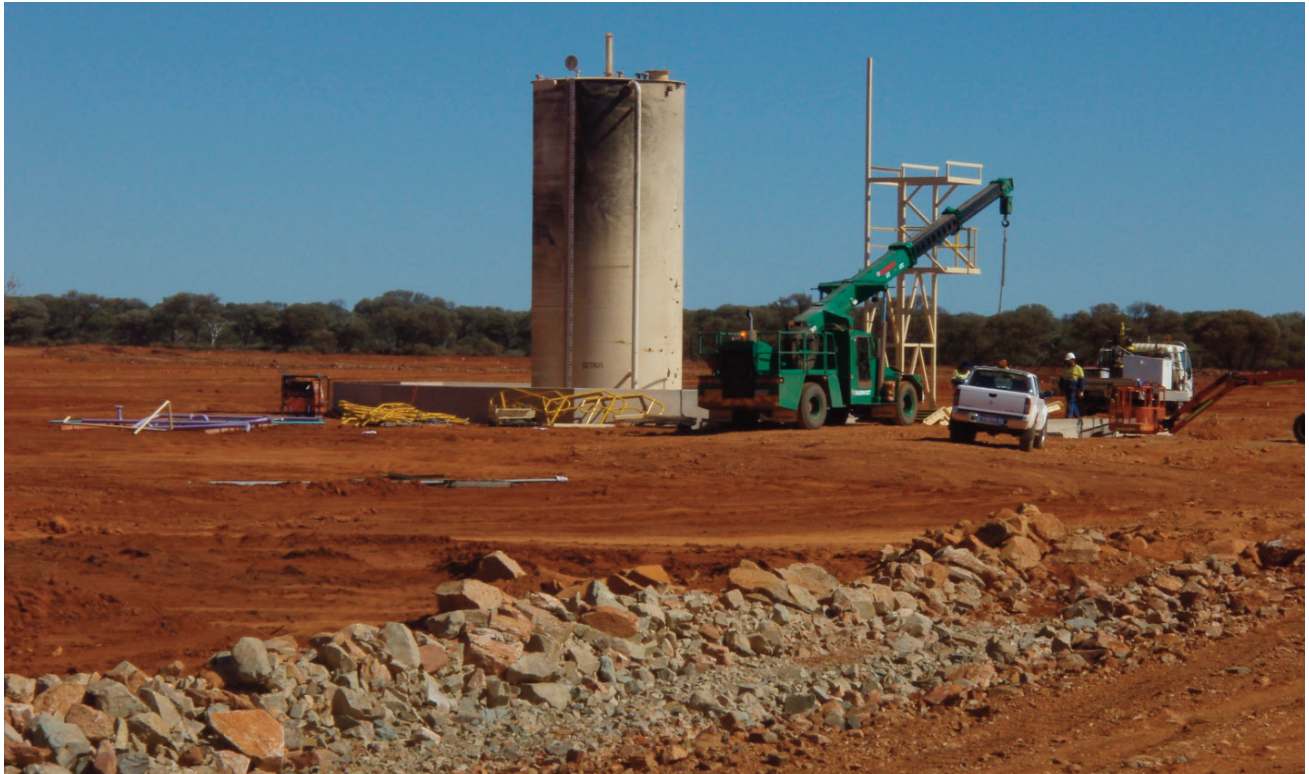
Photo 1. Completed cyanide storage tank installation and concrete bunding.
