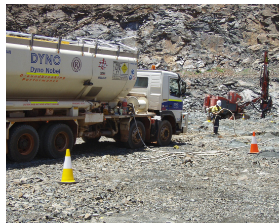
Loading of blast holes
