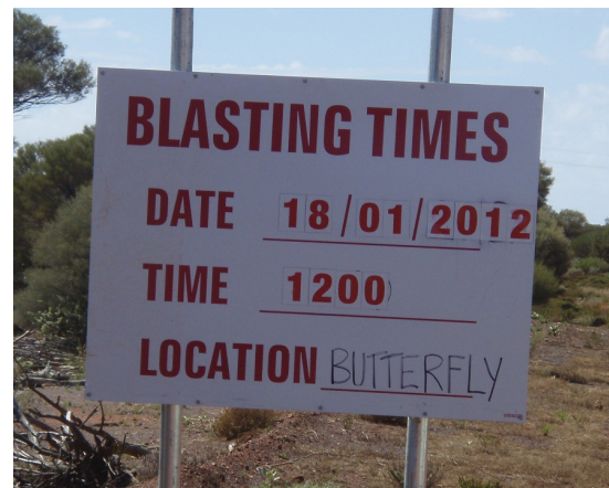
First Blast at Butterfly Pit
