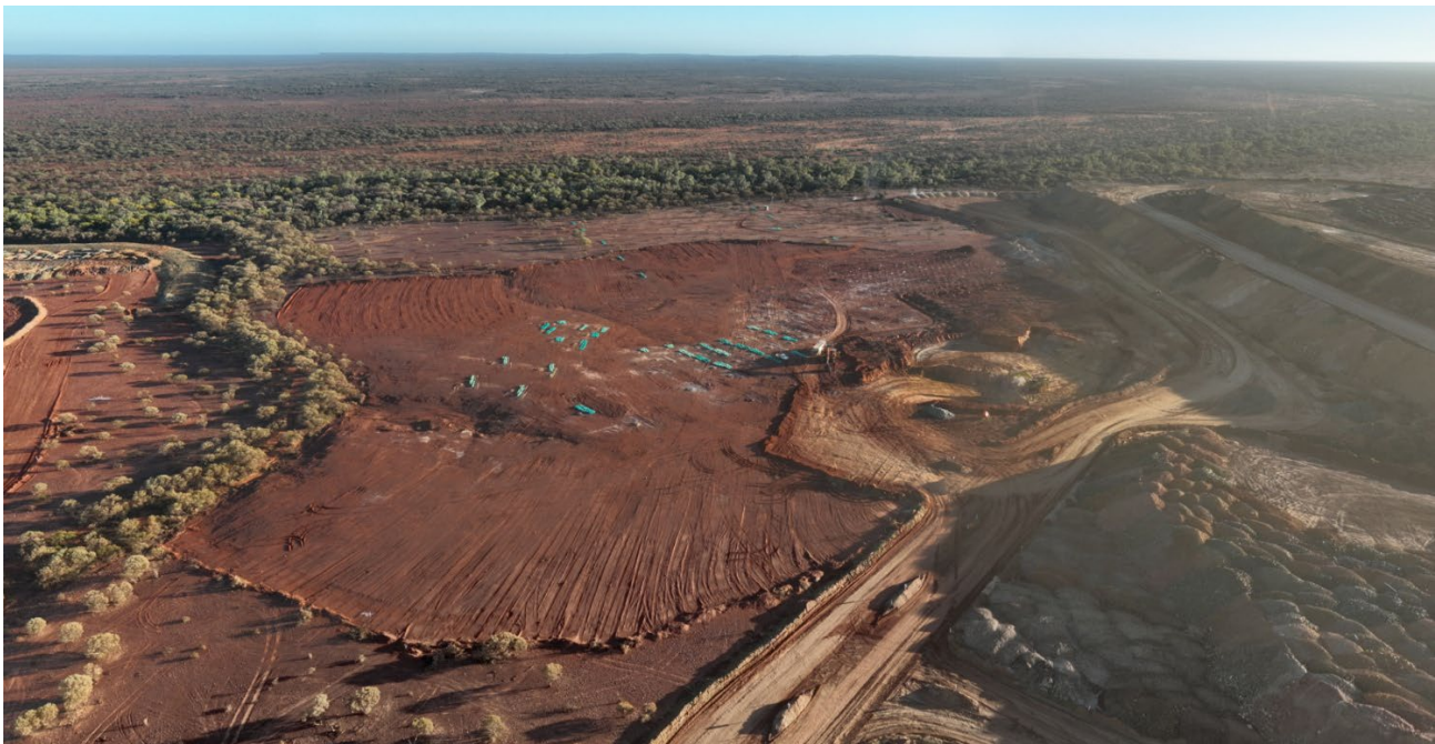
Figure 4: Cloudkicker open pit at the end of June 2026
