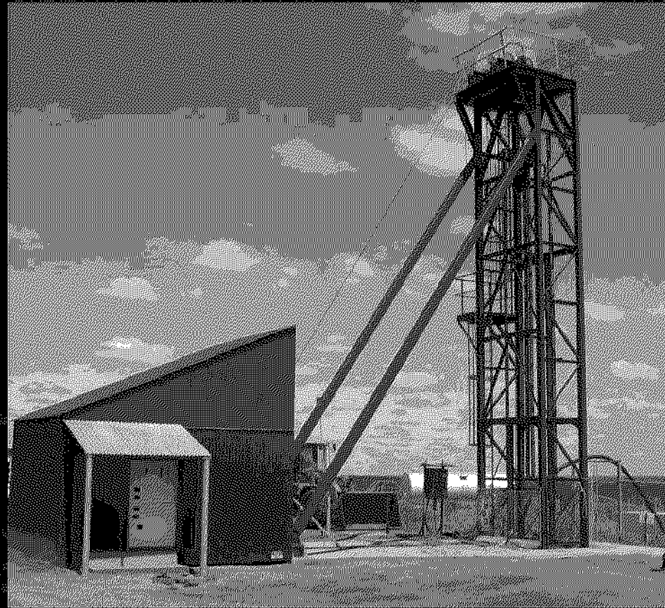
New Headframe Sand Queen Main Shaft
