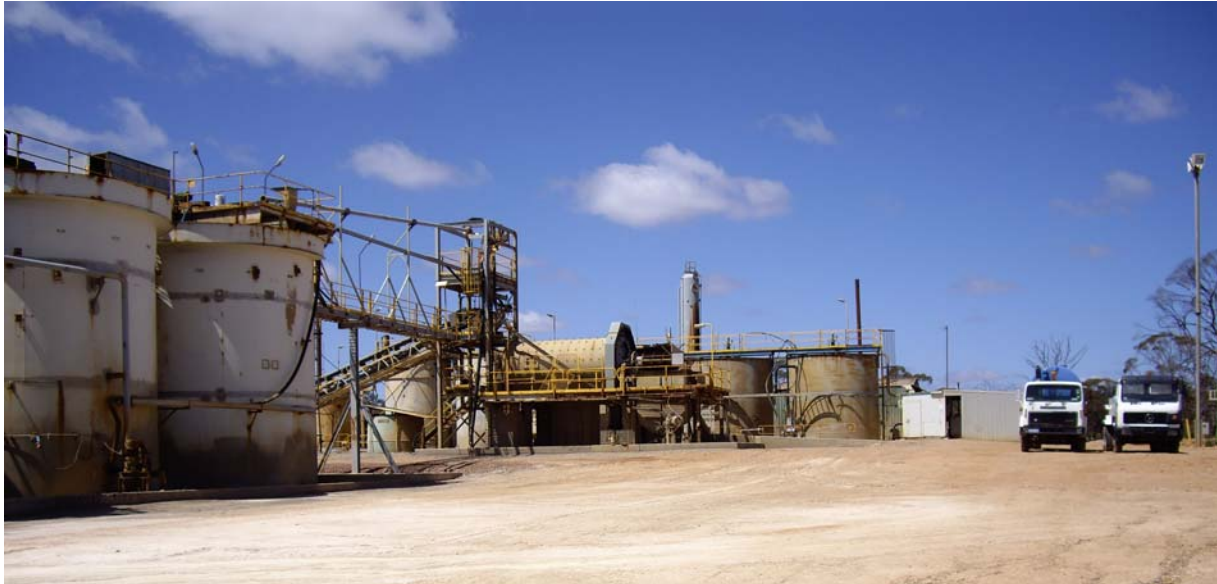
Figure 4 Part of the Nimbus processing plant showing the ball mill (centre) and leaching tanks (photo courtesy PGPL).
