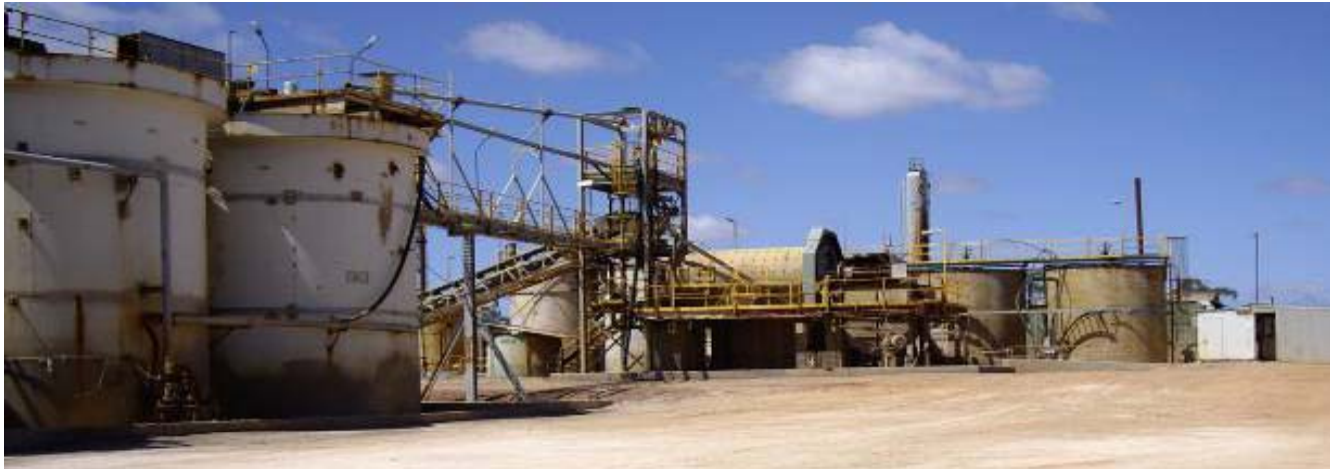
Nimbus Processing Plant
