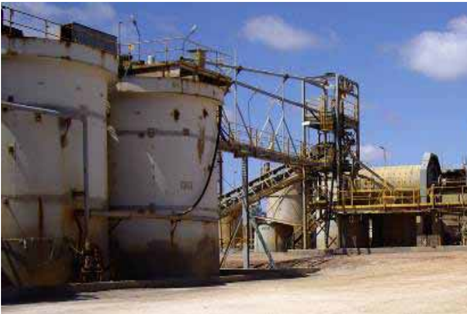
Nimbus Processing Plant
