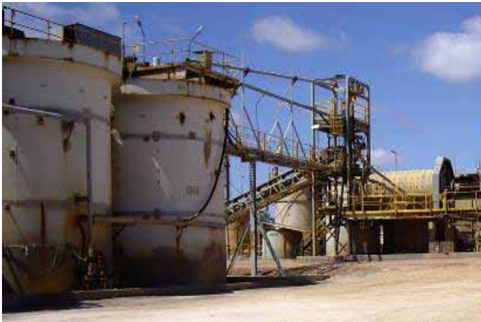
Nimbus Processing Plant
