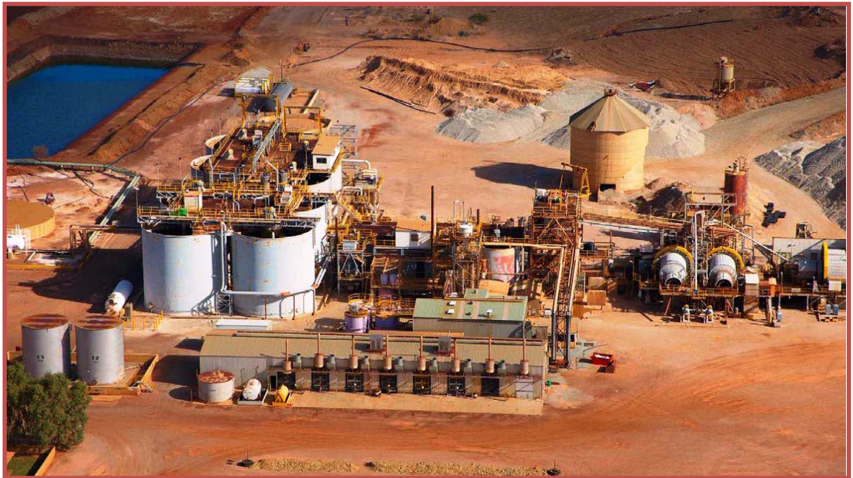
Figure 2 Part of the processing facility at Bluebird, and the power generation plant in the foreground.
