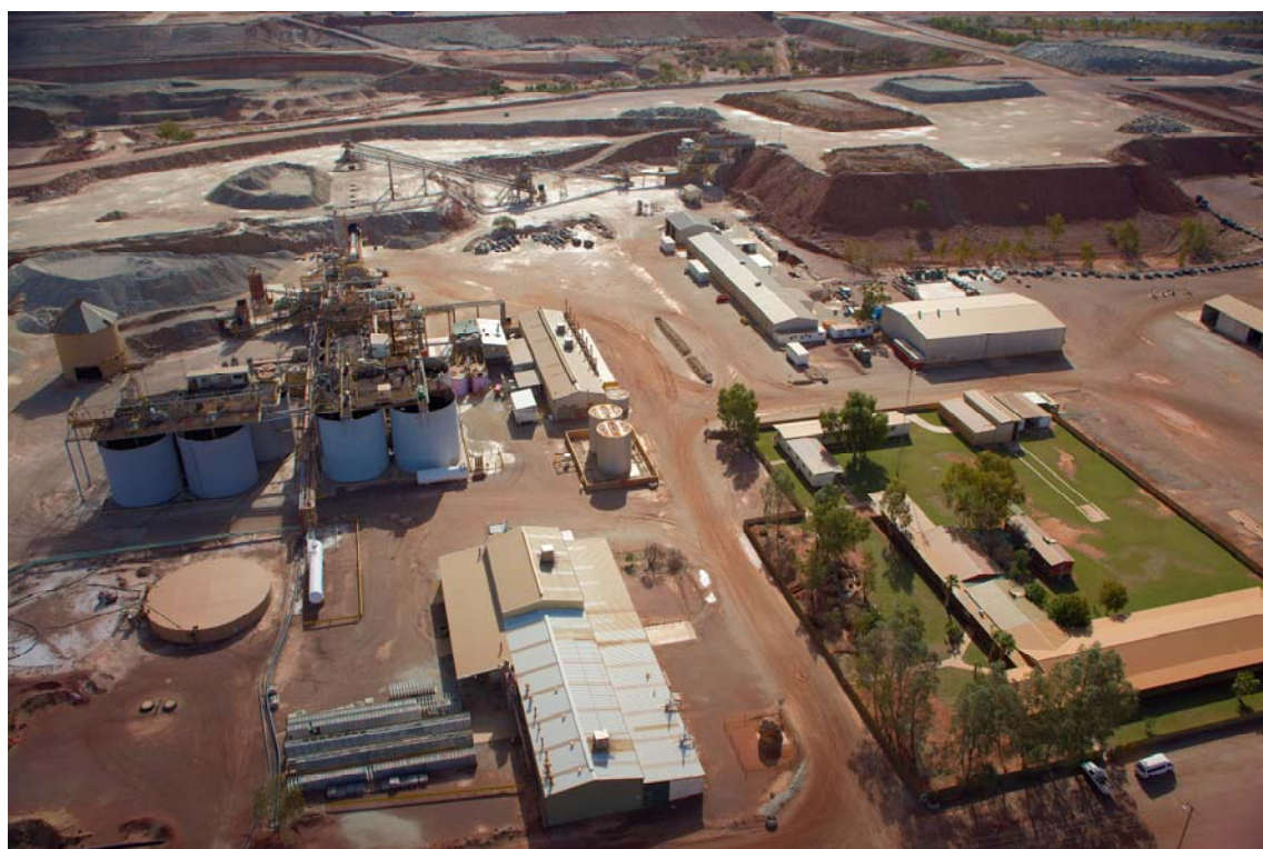
Figure 1 Bluebird Processing Plant
