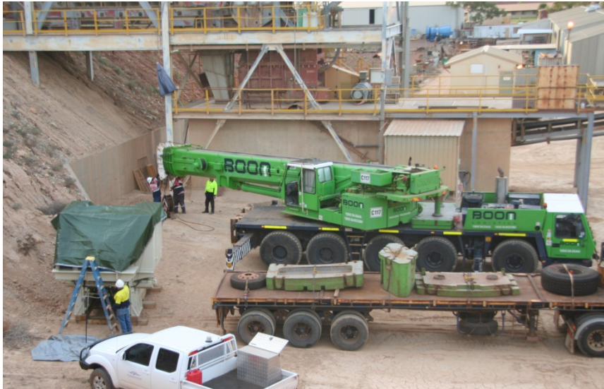
Figure 4. New C125 Primary Crusher arriving on site during the quarter
