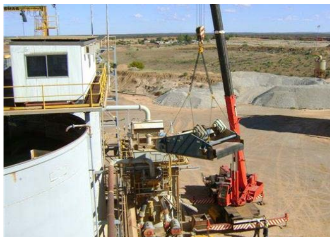
Figure 3. Bluebird Gold Processing Facility tailings discharge screen being removed for maintenance
