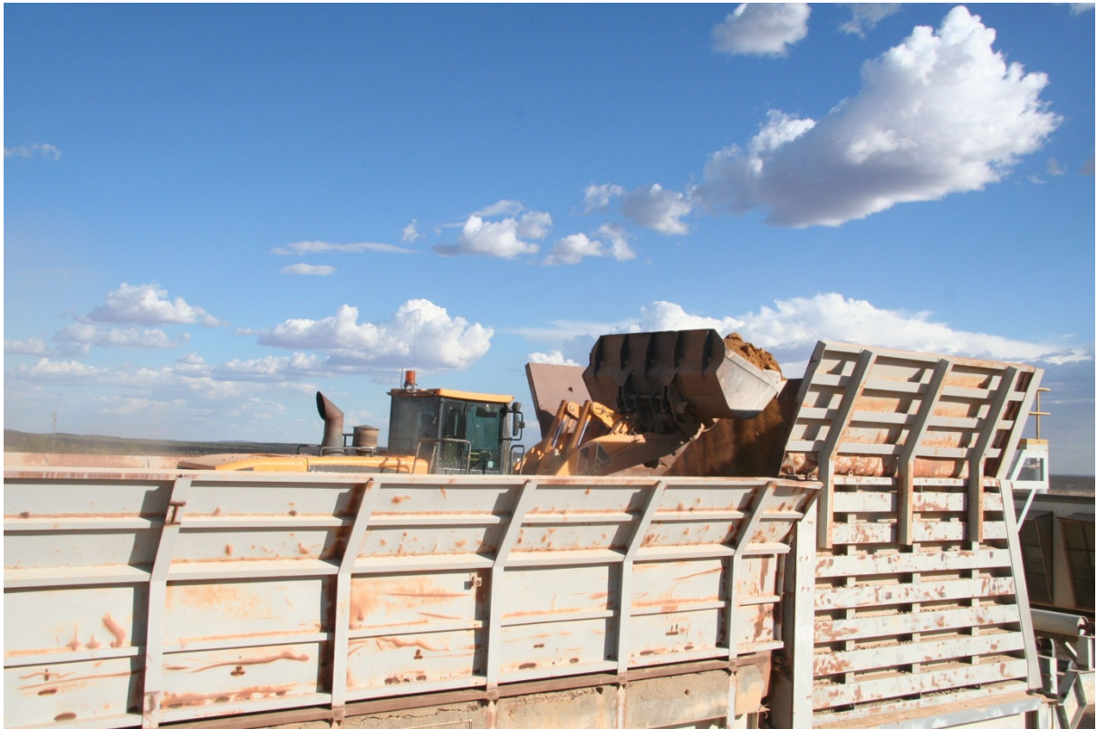
Figure 1 – Run-of-mine stockpiled ore being fed to the Bluebird primary crushing circuit.
