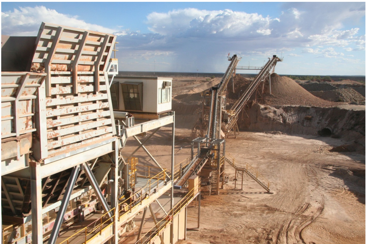
Figure 2 – Crushed ore being stacked on the Bluebird live ore surge stockpiles prior to feeding the plant milling circuit.
