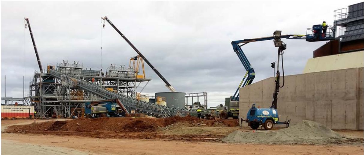
Image 2. Beneficiation Plant under construction
