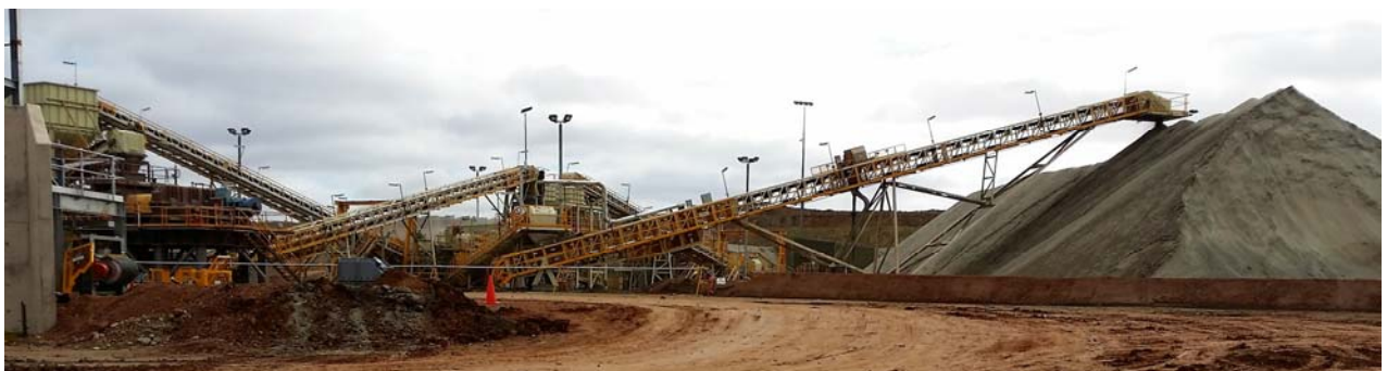
Image 1. 3-Stage Crushing Plant and Crushed ore Stockpile
