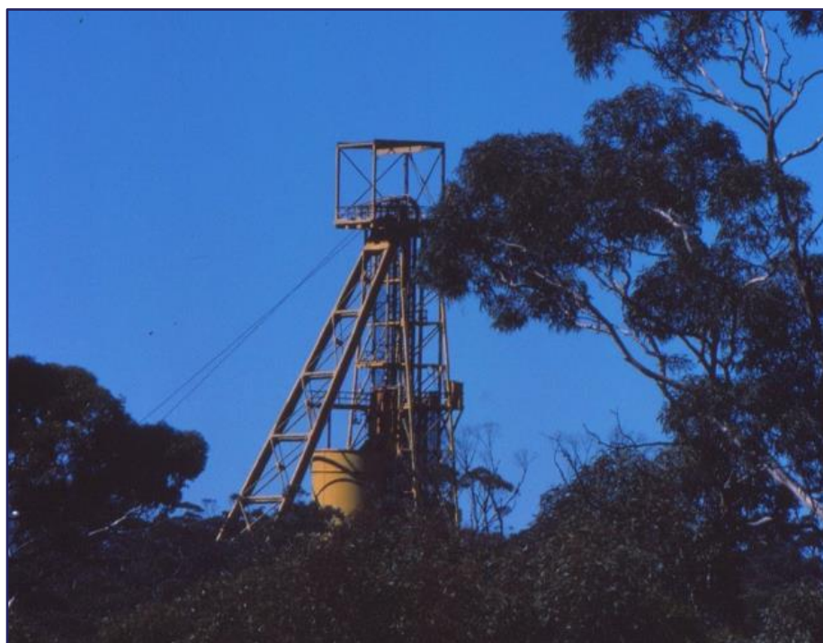
Figure 1 – The headframe over the Mt Edwards 26 North underground mine circa 1990. The headframe has been removed however the shaft remains in place over the residual Mineral Resource (Photo: Stephen Ireland).
