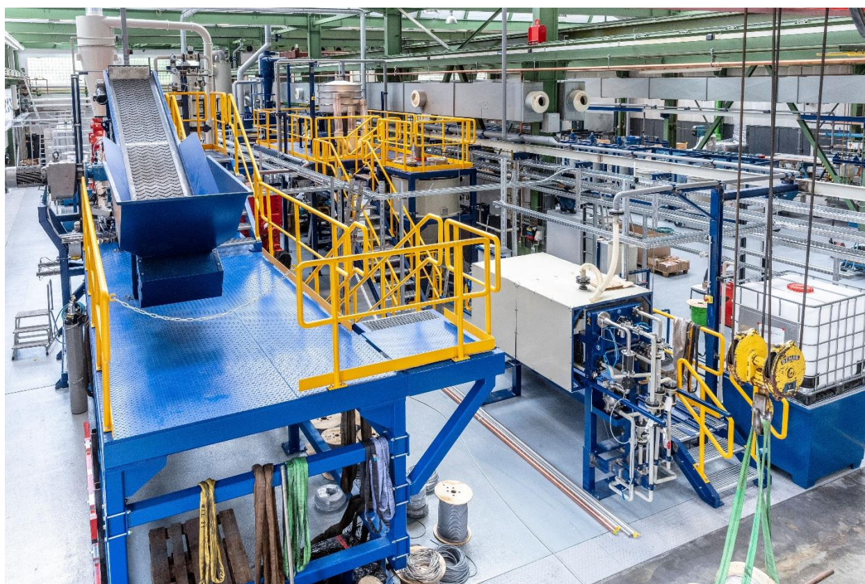
Figure 3 – Two stage Shredding Circuit
