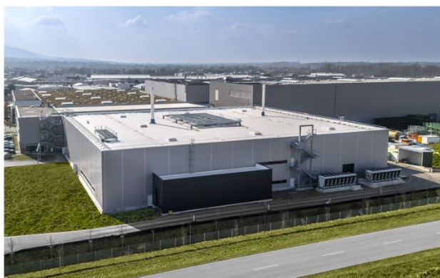
Figure 4 – Mercedes-Benz LiB Recycling Building, Kuppenheim Germany.
