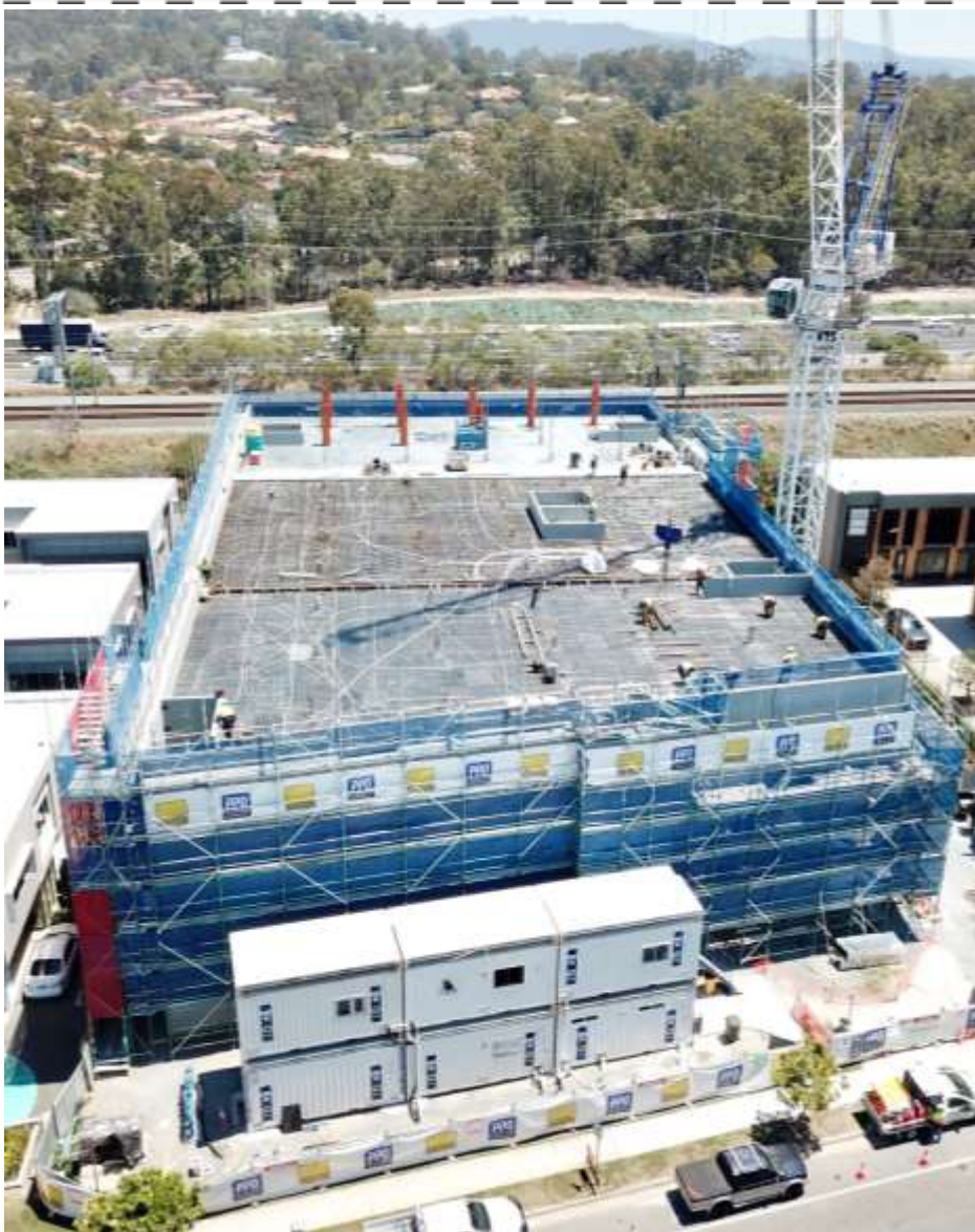
National Storage Robina expansion underway
