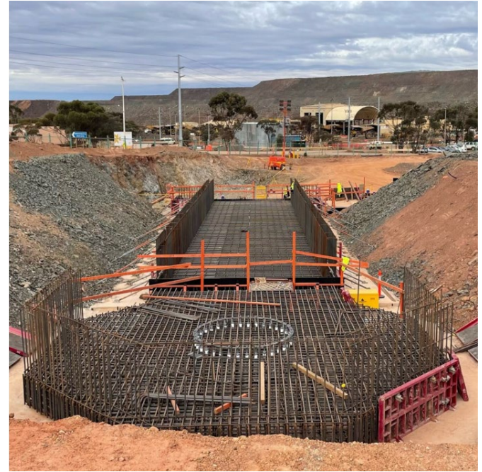
Flotation Thickener Concrete Works
