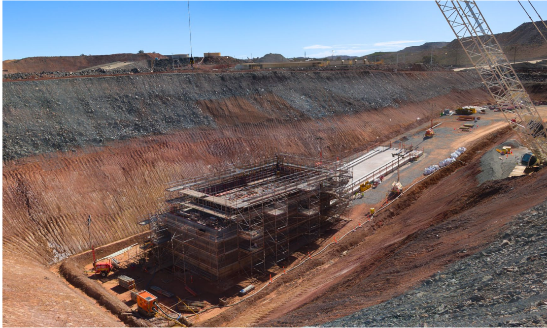
Primary Crushing Area Concrete Works
