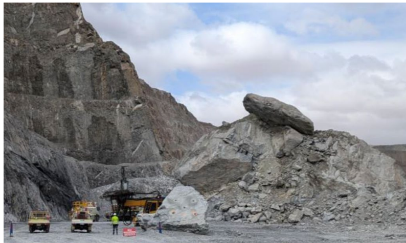
East Wall Remediation
