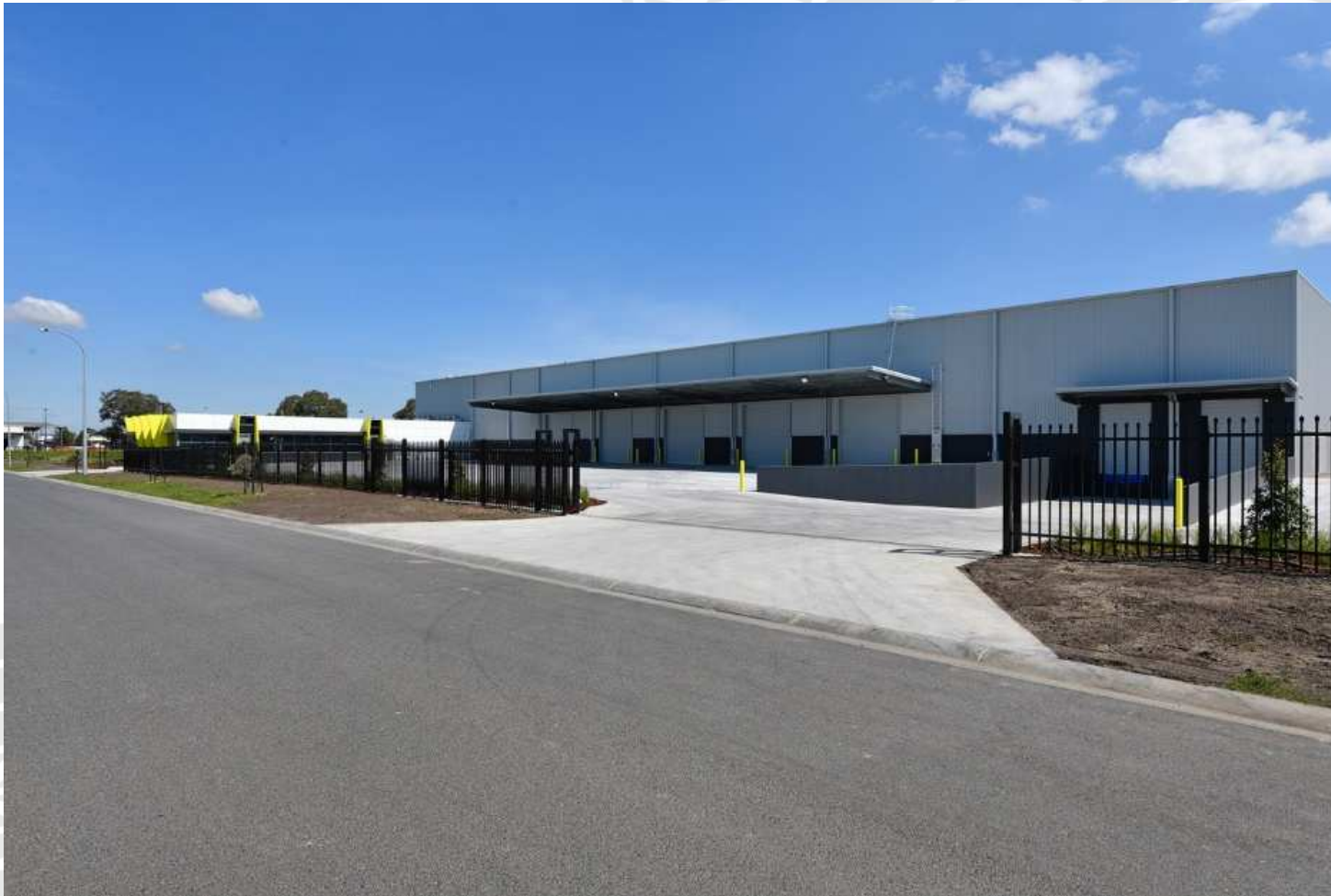
New ETD/Dynamic warehouse Dandenong Vic.
