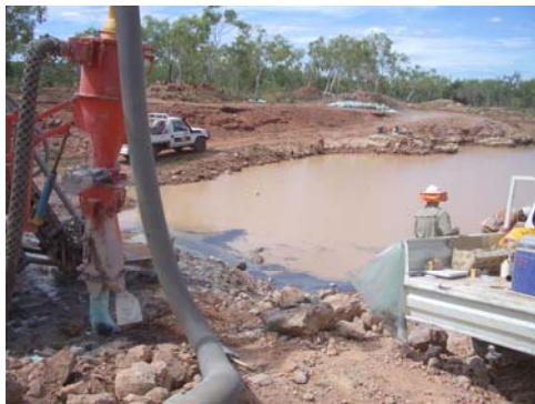
Drilling at Redbank – April 2008
