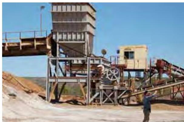
ROM Bin & Crusher
