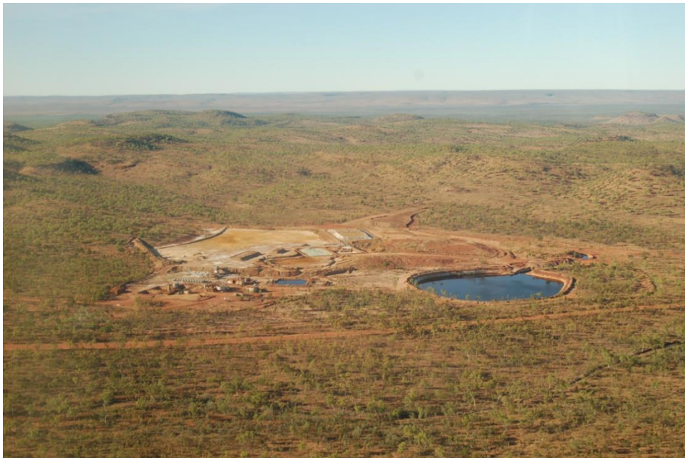
Figure 1. View of the Sandy Flat Mine Site showing the flooded open pit and surface infrastructure
