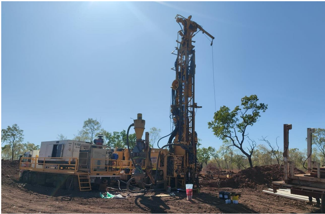
Figure 7: RC drilling continuing at the Redbank Project Airborne EM conductor
