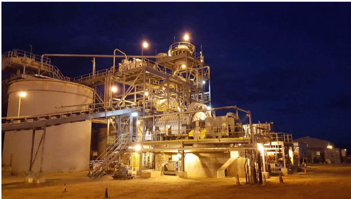
Figure 1: Davyhurst processing plant and equipment now fully operational.
