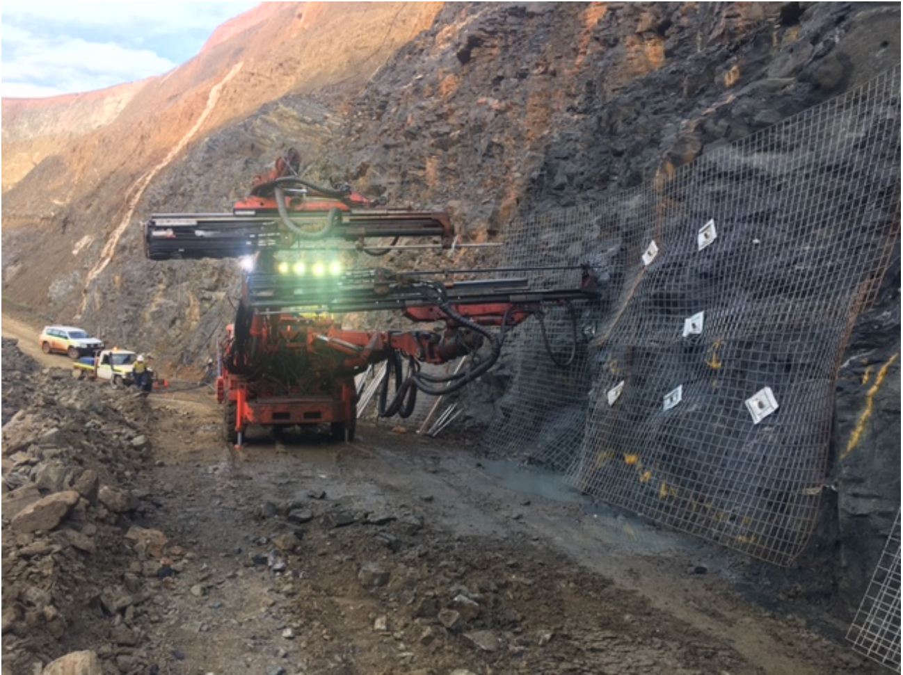
Figure 2: Golden Eagle portal access works underway.
