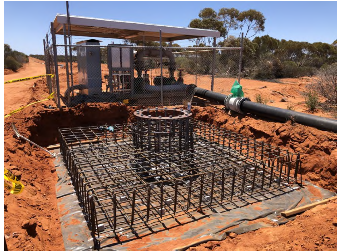
Davyhurst Process Water Supply Footing for Process Water Telemetry Monitoring System Being Installed at Transfer Station
