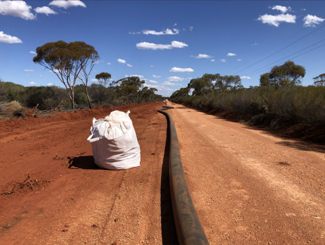
Davyhurst Process Water Supply Process Water Pipeline Firebreaks Re-established and Area Cleaned Up
