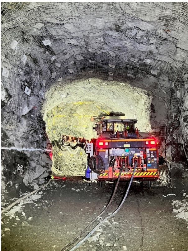
Figure 3 – Jumbo boring out the face on 26 June
