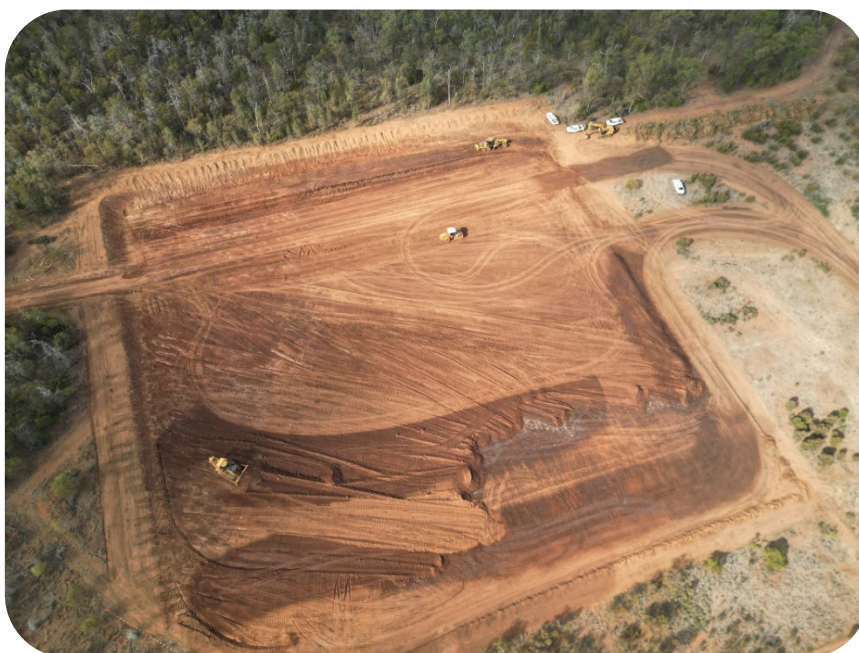
Figure 1: Well-pad preparation
