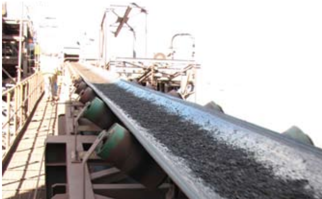
Fines conveyor going into cyclone plant
