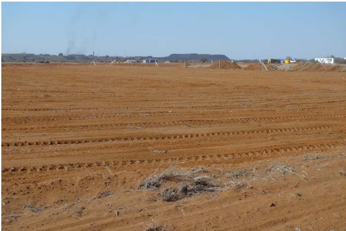
Plant Site Cleared
