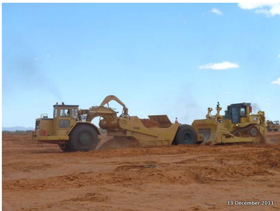
Mine pre-stripping underway
