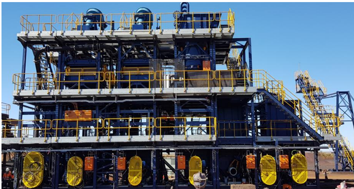
TRP being assembled on site – 11 th July 2019
