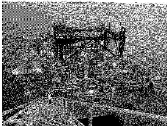
BassGas (Yolla) platform pictured from the flare boom during installation
