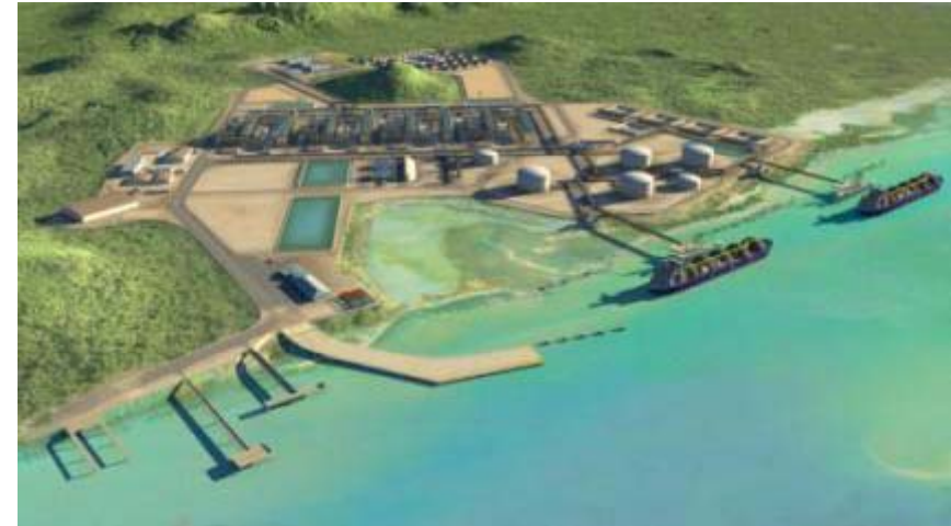
Laird Point (Curtis Island) Picture shows 4 train project
