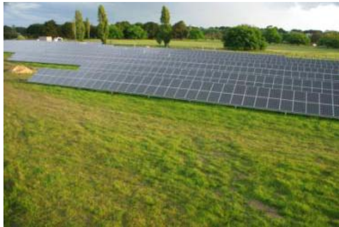
Origin conventional solar panels
