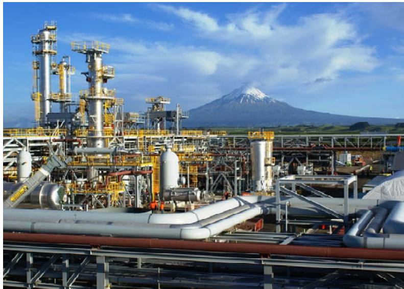
Kupe onshore production facilities
