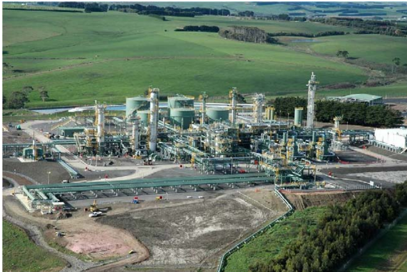
Otway onshore production facilities
