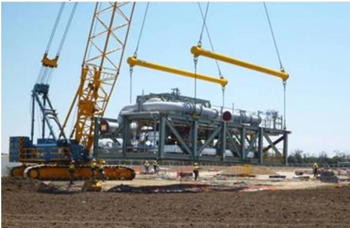
Second Pre Assembled Unit installation at Condabri Central Gas Processing Facility, December 2012
